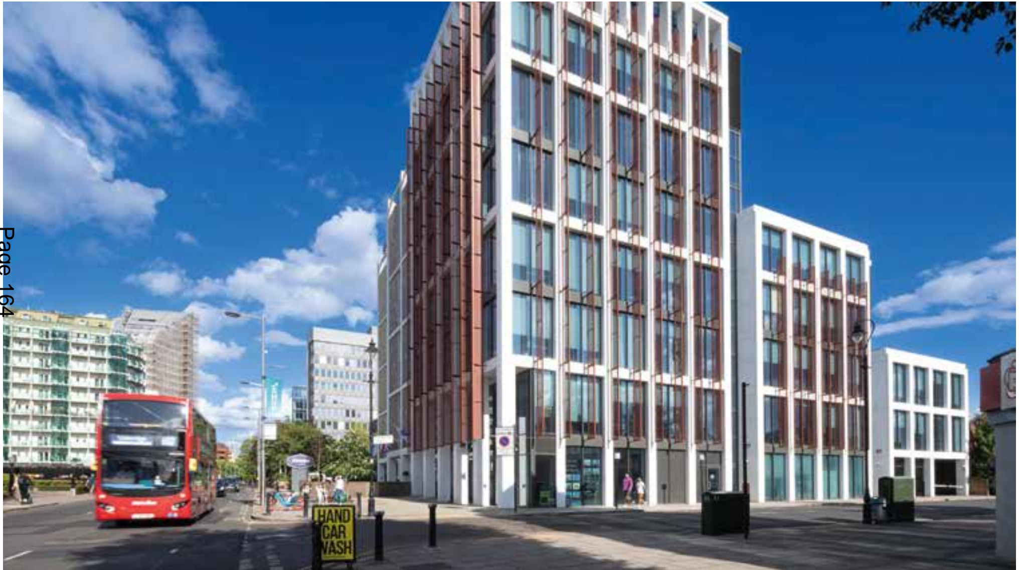
Image: Ealing Town Centre, Uxbridge Road.
