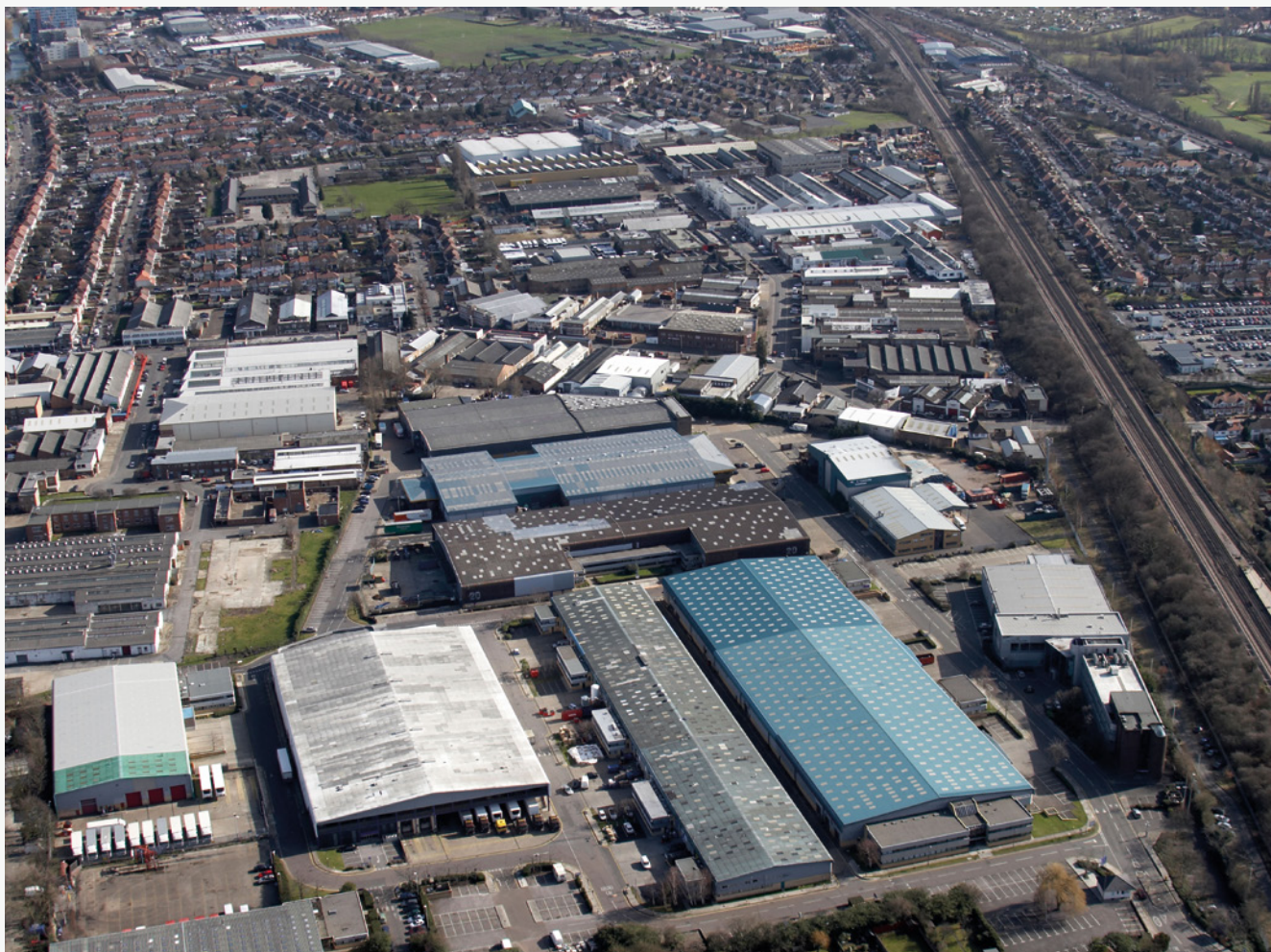
Image: Aerial view of North Acton Industrial Estate.
