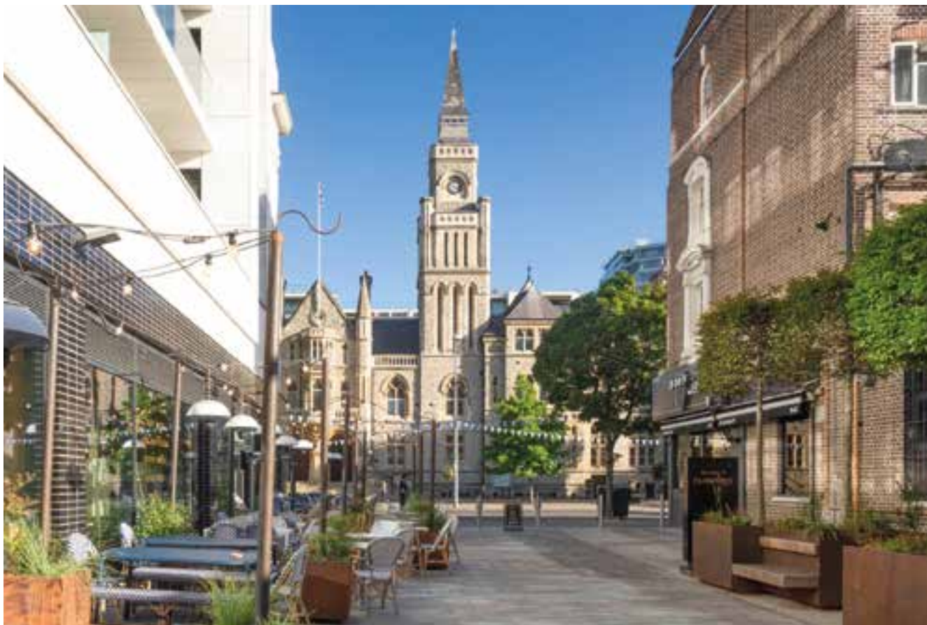
Image: View towards Ealing Townhall from the Filmworks.
