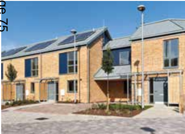
Image: New builds, Britannia Close housing in Northolt, West London.
